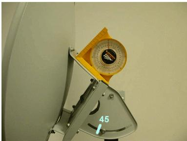
Without any skew adjustment, adjust elevation. You can use an angle locator as shown or use elevation reading on the bracket. (Align the edge of tube to the readings) If you are using a washer on elevation unit, you may not able to see the edge of the tube.
