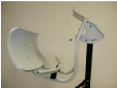
Attach LNBF Guide using B5. Pay attention the orientation of LNBF Guide.
